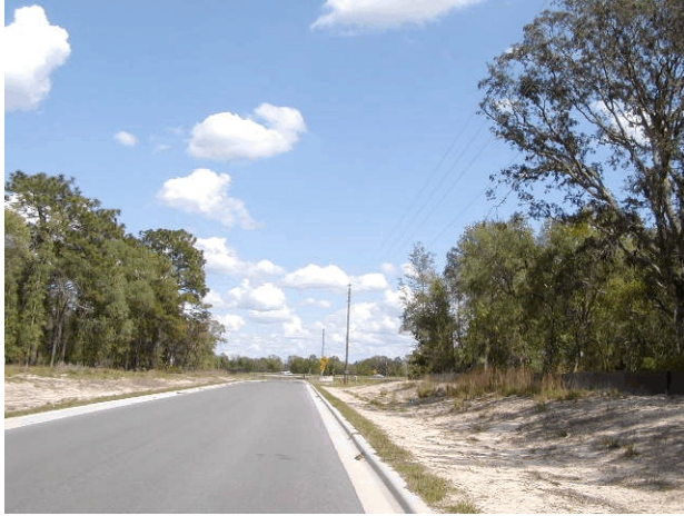
View along Edward Noll Road
