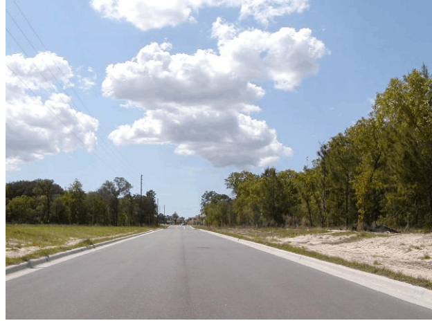
View looking West of Edward Noll Road
